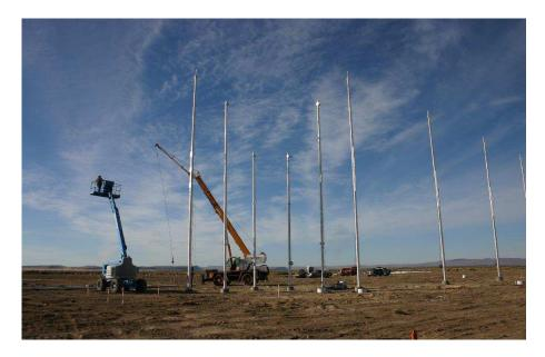
A large crane and heavy equipment were required during the process of erecting the poles. All 64 poles and the tensioning beams were installed in a single, long day. Tensioning and aligning the poles took several more weeks of work by several crews.
