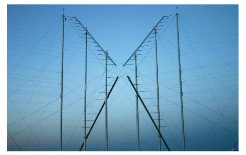
A view of the completed main arrays at the location where the two arrays converge; the Nexus. Guying cable from poles in the adjacent arrays cross in this region forming interesting geometric patterns.
