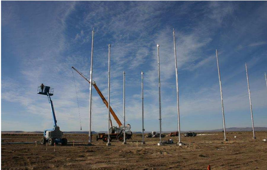
A large crane and heavy equipment were required during the process of erecting the poles. All 64 poles and the tensioning beams were installed in a single, long day. Tensioning and aligning the poles took several more weeks of work by several crews.
