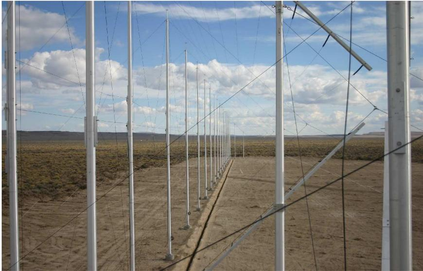
View along East Main array during construction. Visible are aluminum poles, which support the antenna wires and provide tension along the array; Kevlar guying cables; conducting antenna and reflector wires; garage door springs; and a deep, narrow trench where the coaxial cables carrying the RF signals are to be buried.
